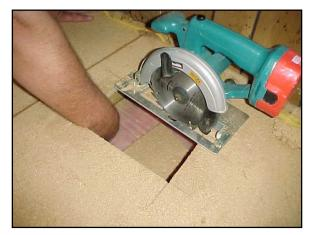
Determine the direction and location of the floor joists. In most cases, the joists run across the width of the home. Generally you will find a joist at the seams of the subfloor. If you're unable to determine the location of the floor joists, cut an inspection hole and feel for the joists with your hand. Again, check to be sure that your floor isn't screwed to1x2's, as mentioned above.
