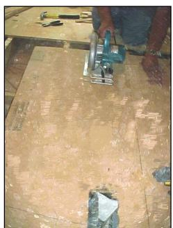
For easiest removal of the old floor, cut down inbetween each floor joists with a circular saw. We prefer to work in sections.
