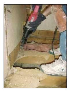
A sawz-all works good for cutting up next to the wall. Be constantly checking for pipes and wires.
