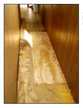
A leaking window was the reason that a large section of the floor in this hallway needed replacing.
