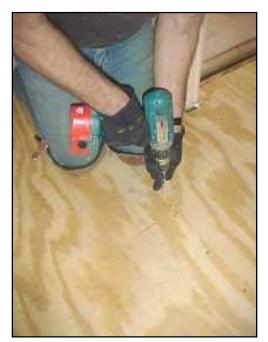
Screw flooring to the floor joists using 2" galvanized screws. Do not nail flooring.
