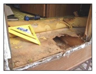
Common places for soft spots is in front of windows and doors. In the repair to the left, the door was removed which made for a solid floor repair job.
