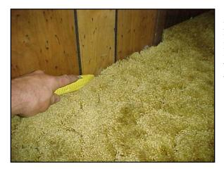
First remove the existing floor covering. In many older homes, the carpeting is layed underneath the walls. So to remove the carpeting, it must first be cut along the walls with a utility knife.
