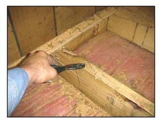
Clean up the top of the joists by removing all the staples and nails. If the old floor was glued, then scrape away any remnants stuck to the joists by using a chissel. Take the proper time and do a good clean job.
