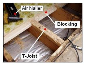
Notice how some of the joists look wider than others. This is called a t-joist, and some factories use these at all the seams. The top of the tee is a strip of subflooring about 3" wide. If this strip appears in good shape, leave it. Otherwise, replace it to keep all the joists the same level.
