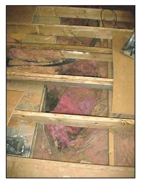
With the floor opened up, this is a great time to beef-up the insulation underneath. Also do any minor belly repairs. When adding insulation, do not smother any waterlines. Keep any added insulation underneath the waterlines so heat from the floor can reach the lines.
