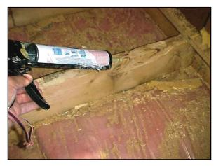
After measuring and cutting the new flooring, construction adhesive should first be applied to the tops of all the joists. This will help minimize floor squeaks.
