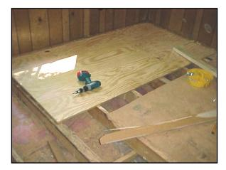
After applying the adhesive, lay down the first piece of plywood flooring and screw into place using 2" galvanized screws. Screws are preferred over nails as they are less likely to pop.
