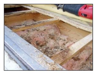
IMPORTANT NOTE: In some rare instances, your subfloor may not be screwed directly to the floor joists, but instead screwed to 1x2's nailed across the floor joists. Inspect for these before doing any cutting. You DO NOT want to cut the 1x2's.
