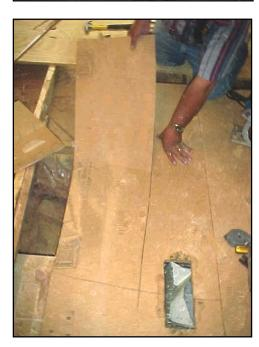
Pull up the cut pieces and throw out the window into the dump trailer. If the flooring is glued to the joists, the pieces may not come up easily.
