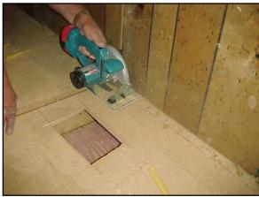
If replacing the floor along a wall or an entire room, cut along the edge with a circular saw. To cut, we put the saw guide against the wall and cut. This left 1" or so of old flooring. If the old flooring isn't rotten around the edges, this may be OK.
