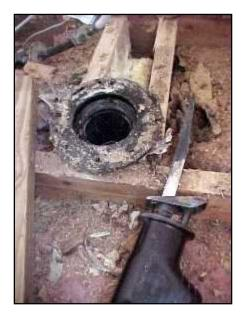
Replacing the floor underneath a toilet generally involves cutting off the toilet flange, and installing a new one after the new floor is installed. See our 30 minute how-to video for more details.
