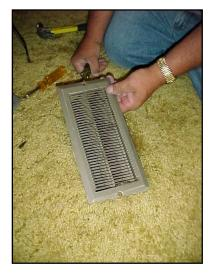
Also remove the floor registers. Most are taken out by removing two screws and then prying up.
