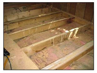
The first section is now ready for new 3/4" plywood subflooring. Laying the floor in sections may be easier than ripping out the whole floor at once. Plywood offers much greater strength than partical board.
